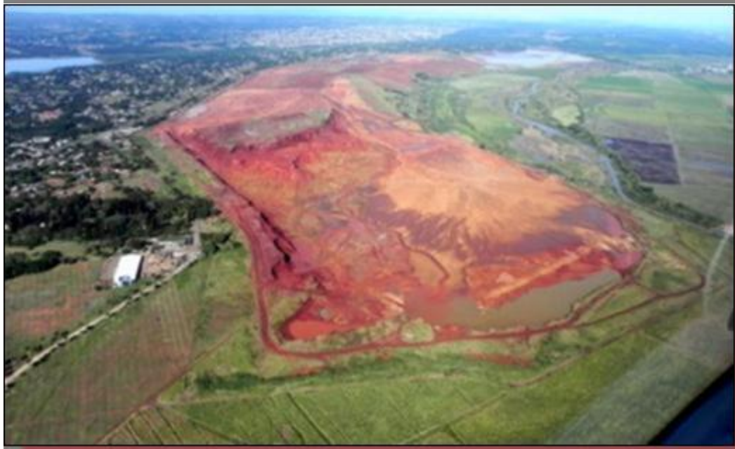
Exxaro KZN Sands Hillendale mine next to UVS and Ezikaweni settlements. This is what it will look like south of Mtunzini, and east of the N2 if the mine goes ahead.
